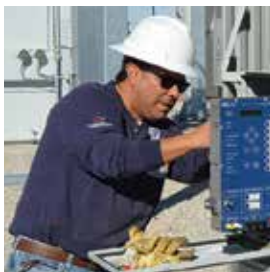
MARCOS MARTINEZ Substation Tech 20 years
